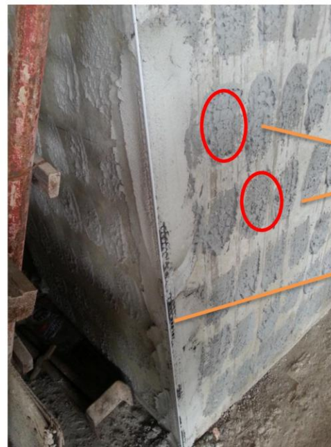
Insert corner beam and splash dash. Function of splash dash is to enhanced griping power of Ordinary Portland Cement (OPC).
