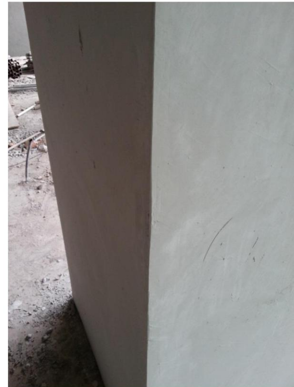
Smooth and even surface after drying.
