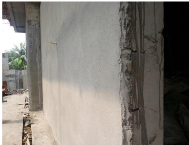
Finishing wall with OPC.
