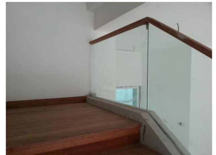
Finished baluster and handrail.
