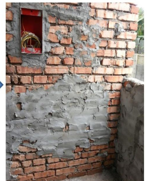
Plastering the wall
