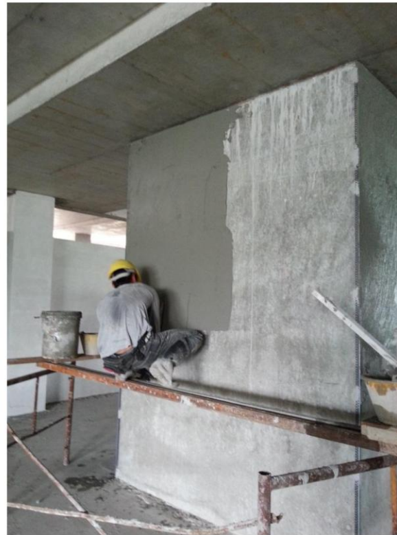
Worker applying Thin Render on the wall.
