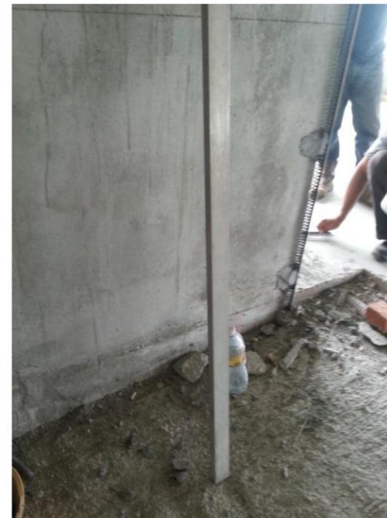
Worker applying Thin Render on the wall.
